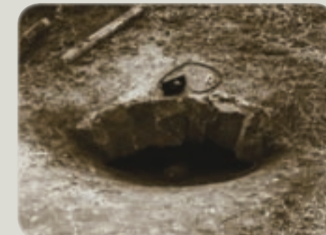
Above: North end of the Law Tunnel in the 1950's, almost completely hidden under allotments. Photo: Copyright © Elliott Simpson
