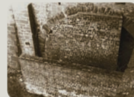
Above: South end of the Law Tunnel with blast walls built during its time as a wartime air raid shelter. Photo: Copyright © Elliott Simpson
