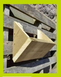
12. Reposition the shelves over the battens and drill two pilot holes through each side of the shelf at top and bottom. Be careful to avoid the screws already there!
