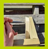
10. Cut the batten along the pencil line, and repeat to make four batten supports. These will butt up against the inside of the shelves as shown (left). Mark the position of each batten on the backing with pencil.
